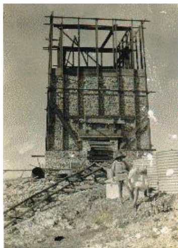
The Memorial at about one-third construction – note small rail line for spawled stone conveyance on left, tool shed and water tanks used during construction.
